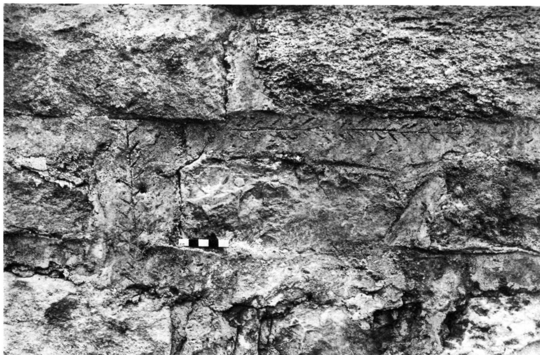
Plate 10 Inmost Ward 1977: Detail of pointing on north (landward) face of late 4th-century riverside wall showing incised herringbone design (5cm scale).
