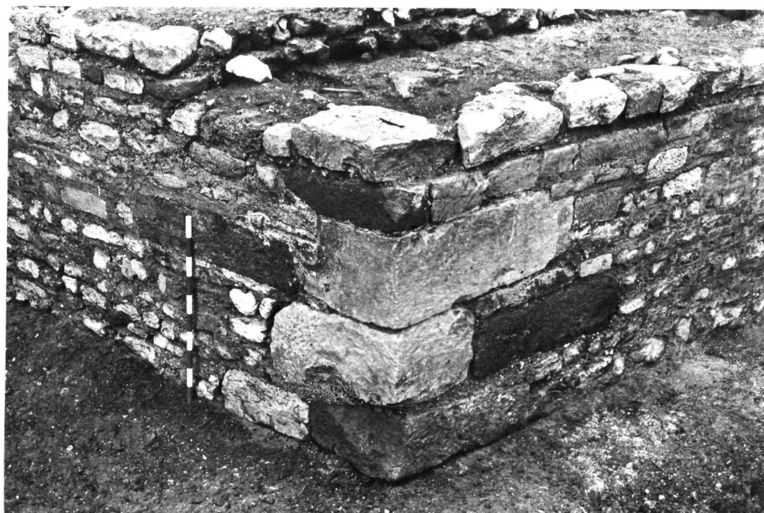
Plate 7 Inmost Ward 1977: Angle of late 4th-century riverside wall showing reuse of architectural stone (1m scale).
